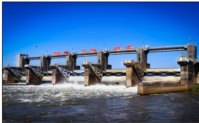
Figure 2: John C Stennis Lock & Dam [14]
