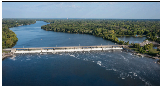
Figure 3: Coon Rapids Dam [13]
