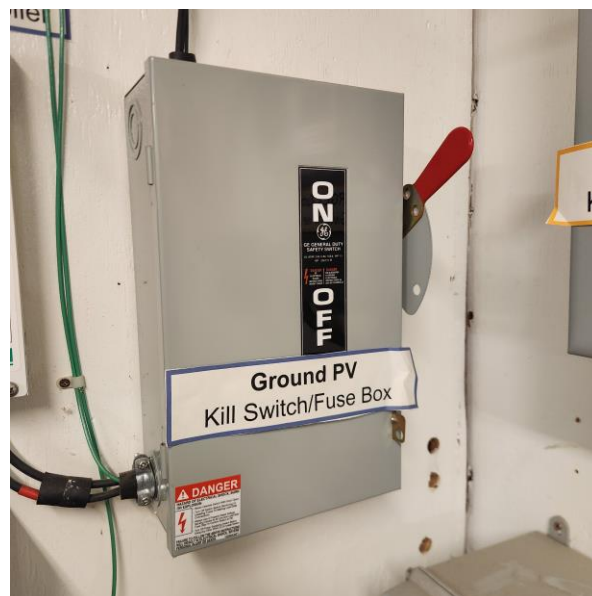
Figure 5: Ground PV Killswitch in the “ON” Position
