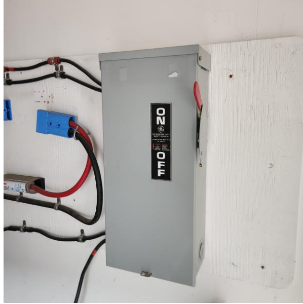
Figure 6: Battery Killswitch in the “ON” Position
