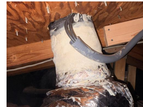
Figure 13: Air Duct Sealant
