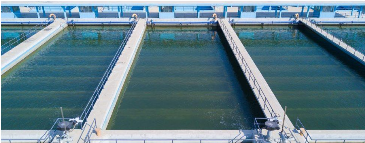
Figure 7: Rapid Sand Filter Example [a]
