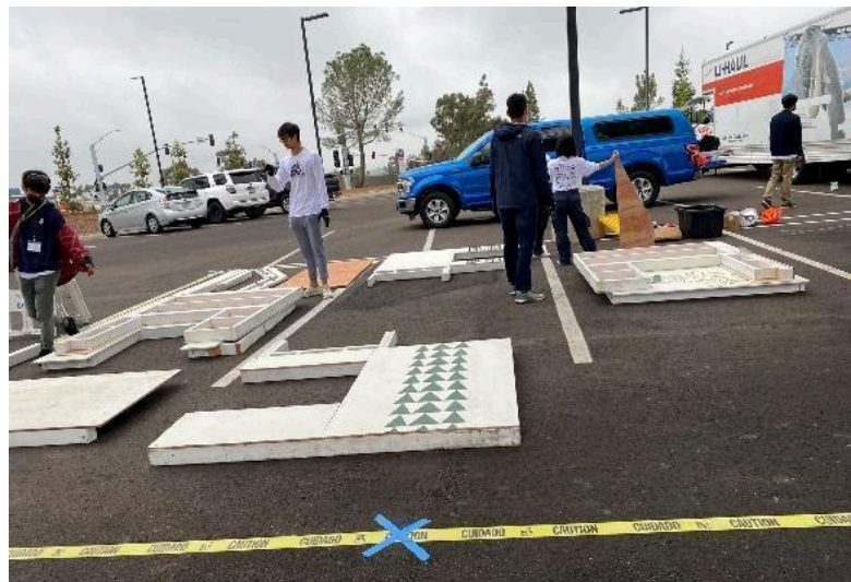
Example of panelized walls at 2022 TSDB
