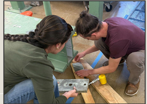
Figure 15: Truss plate installation
