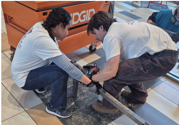
Figure 50: Display Day Construction, North Side [16]
