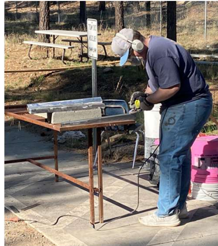
Figure 47: Grinding Down Rusted Members [15]
