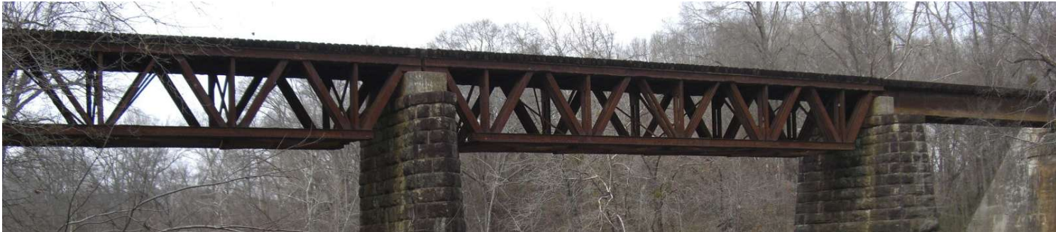
Figure 4: Underslung Truss Example [3]
