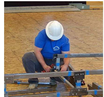
Figure 56: Connecting Bottom Cords [16]
