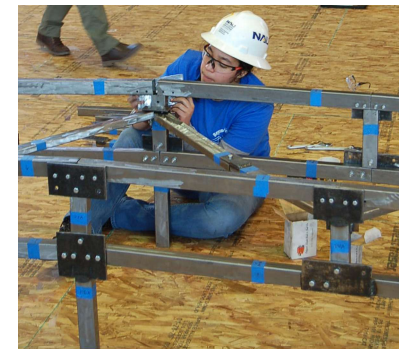
Figure 57: Connecting Members with Plates [16]
