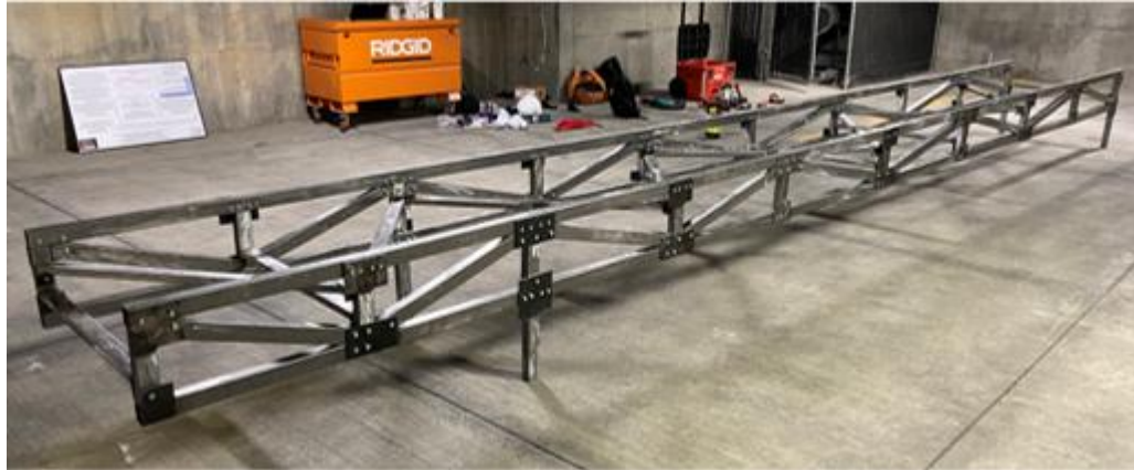
Figure 7-1: Completed Practice Build of Bridge
