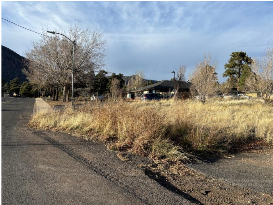
Figure 2-4: Culvert and Gravel Road
