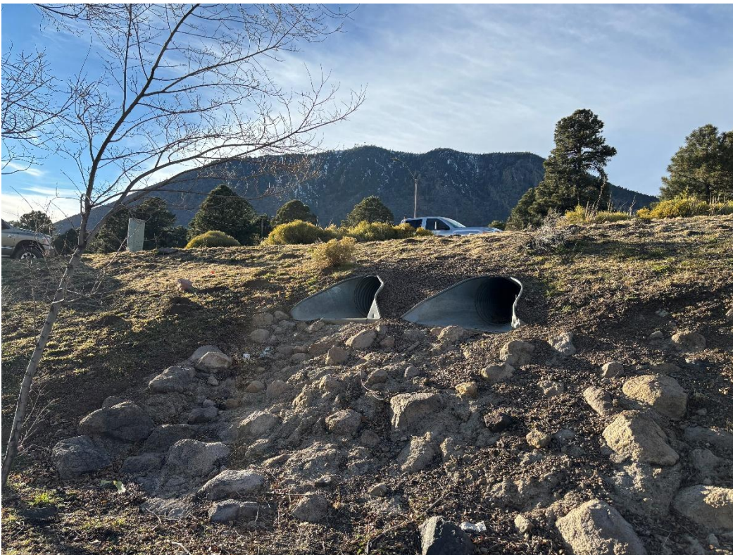
Figure A- 4: Existing Culvert Conditions Downstream of Hwy 89
