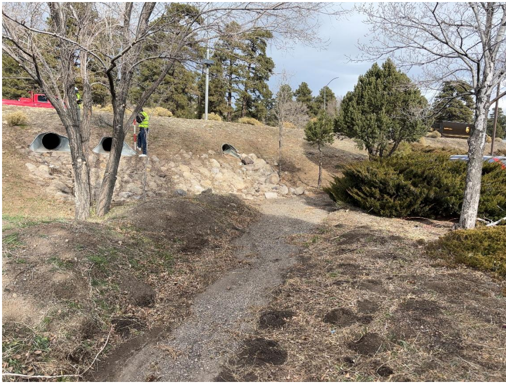
Figure A- 2: Existing Conditions Downstream of Culverts
