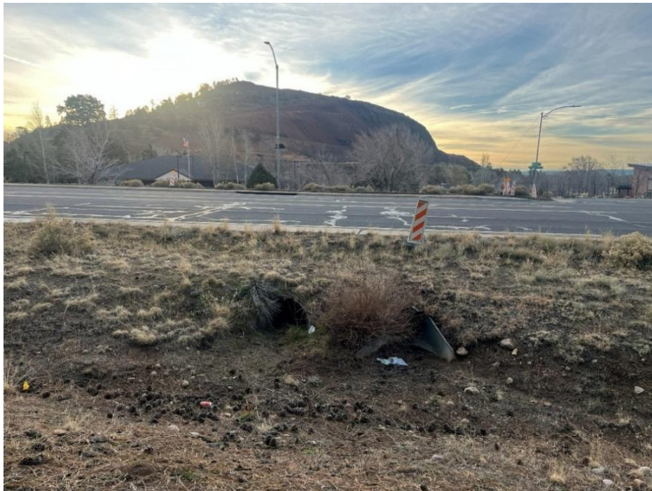
Figure 2-2: Upstream of Site Showing Double Barrel System Under Hwy 89
