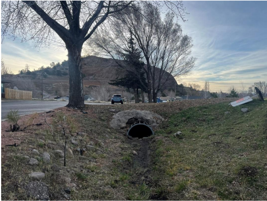
Figure 2-3: Culvert Inlet Under Forest Service Parking Lot
