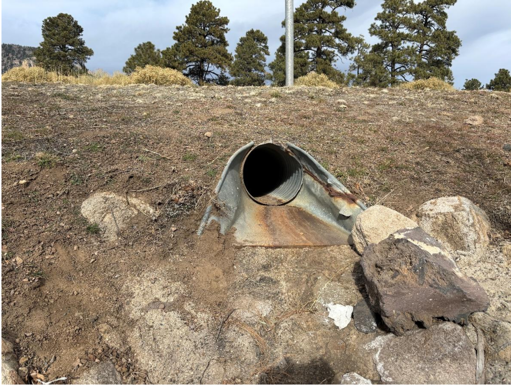
Figure A- 3: Current Conditions Downstream of Hwy 89
