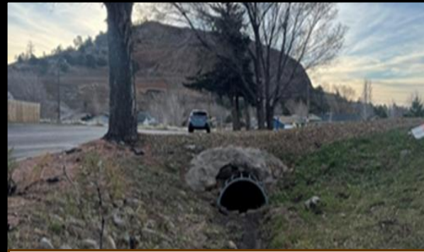
2 Culvert Under Parking Lot
