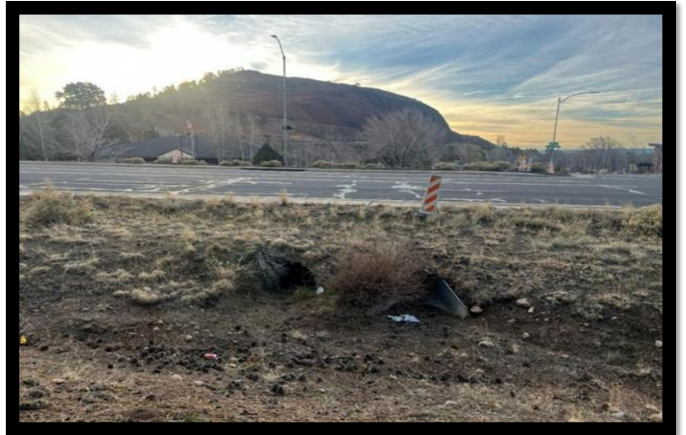
Figure 16: Upstream Side of Highway 89 Culvert
