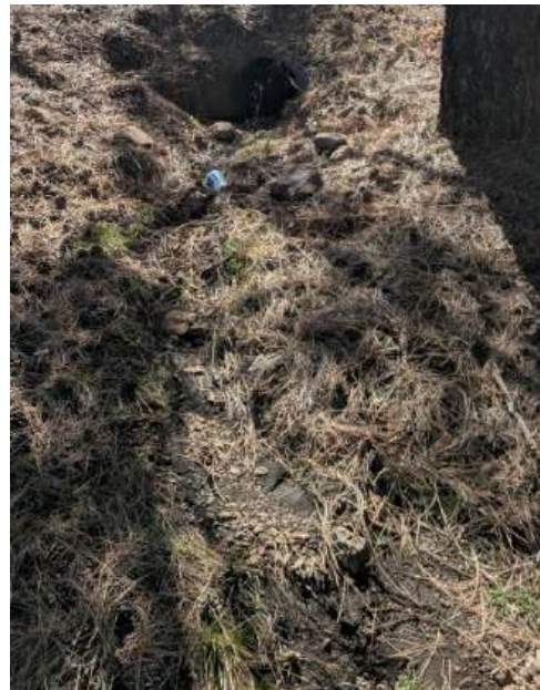
Figure 10: Parking Lot Culvert Outlet Channel
