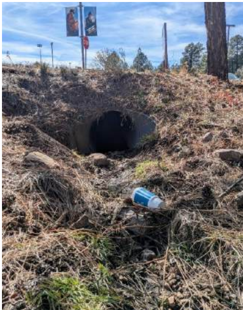
Figure 9: Parking Lot Culvert Outlet
