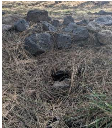
Figure 15: Trail Culvert Outlet
