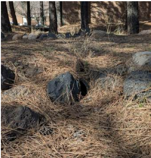
Figure 14: Trail Culvert Inlet
