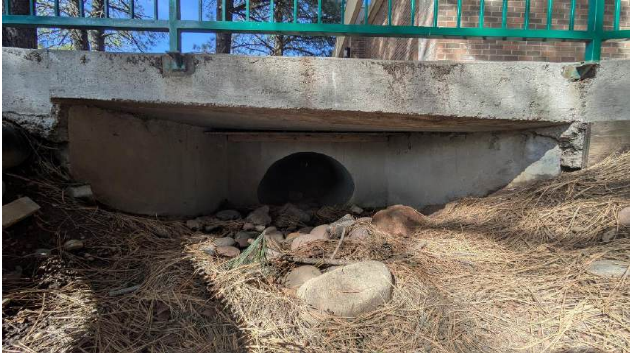
Figure 13: Culvert Inlet
