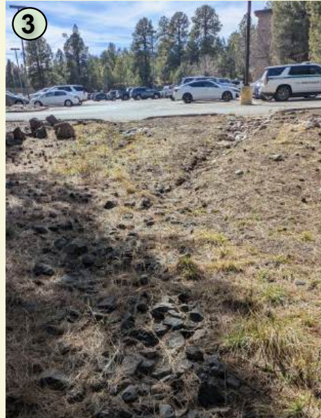
Figure 30: Parking Lot Curbcuts
