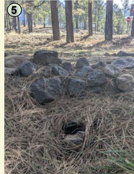
Figure 1: Culvert Beneath Trail
