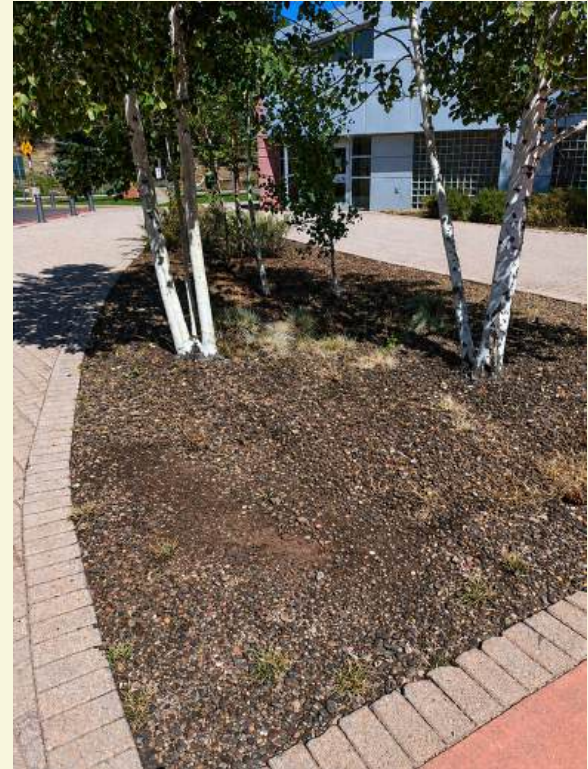
Figure 2: Example of Poor Location
