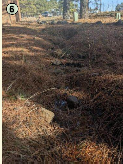
Figure 25: Inlet Channel Erosion
