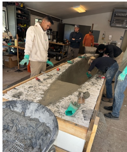
Figure 4-7: Final Concrete Placement
