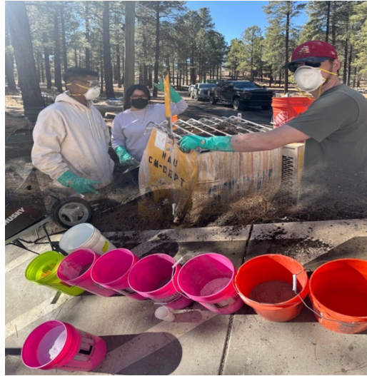
Figure 4-6: Concrete Mixing Process
