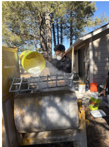
Figure 2-3: Concrete Batching
