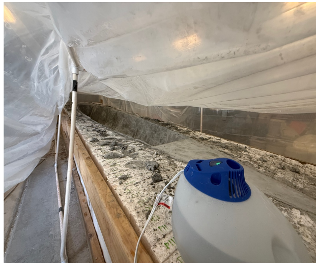
Figure 4-10: Concrete Canoe Curing
