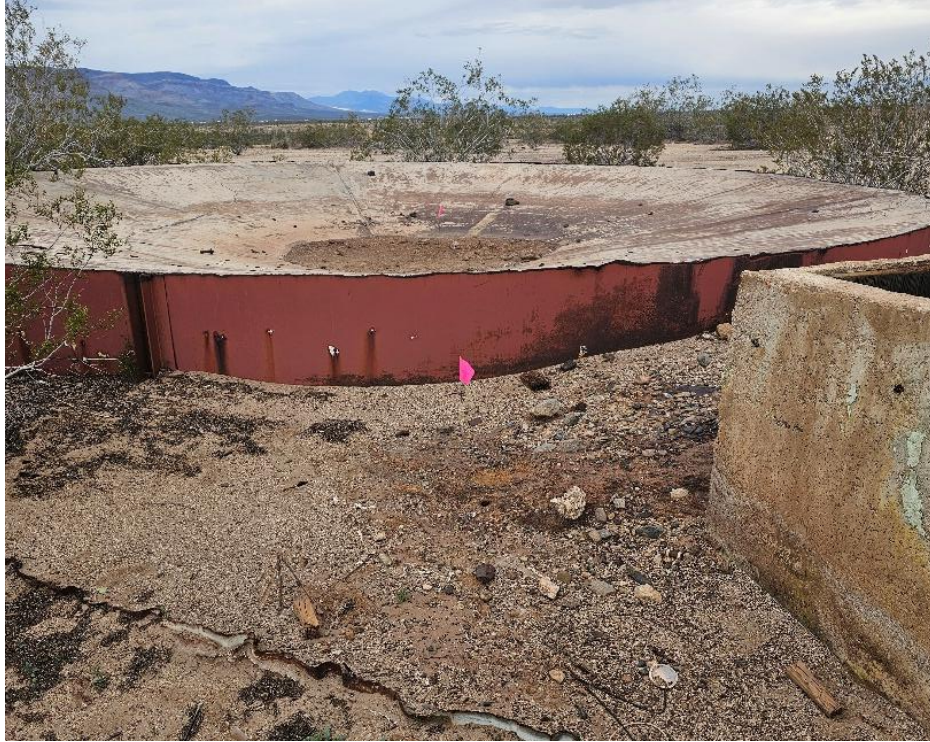
Figure 3.3: Red Concrete Basin (credit: Rashel DeLeon)
