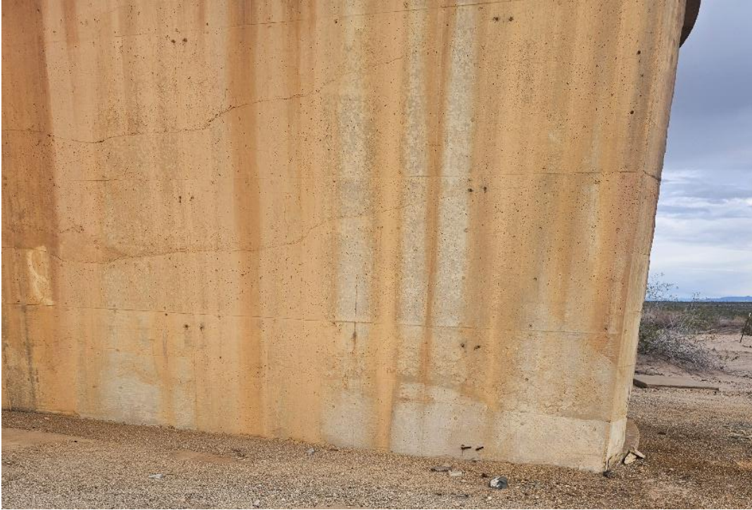
Figure 3.9: Side View of the Orange Building (credit: Rashel DeLeon)
