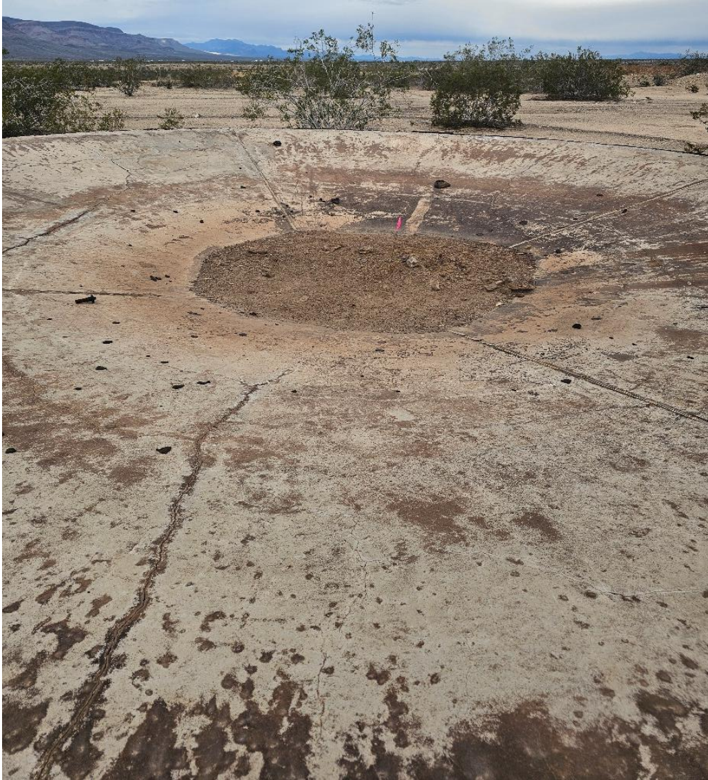
Figure 3.5: Close-Up of Concrete Basin (credit: Rashel DeLeon)
