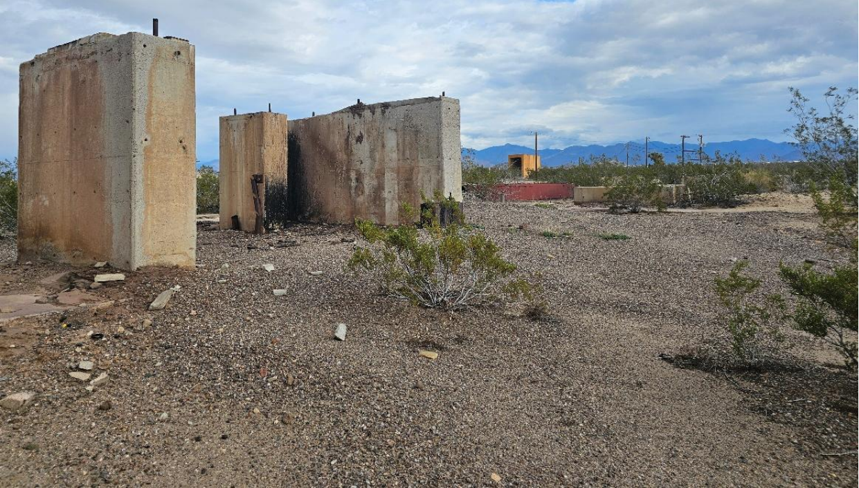
Figure 3.2 Various Mill Structures (credit: Rashel DeLeon)
