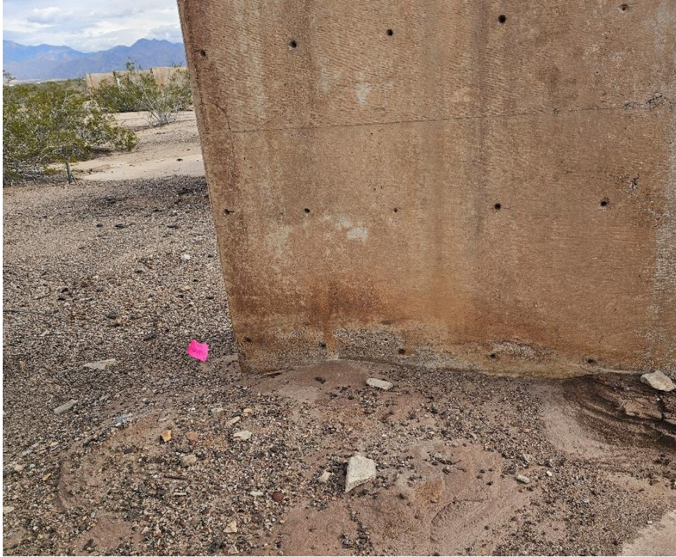
Figure 3.7: Concrete Wall Close Up (credit: Rashel DeLeon)
