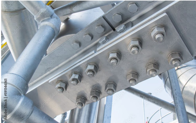
Figure 22, Example Bolted Connection [12]
