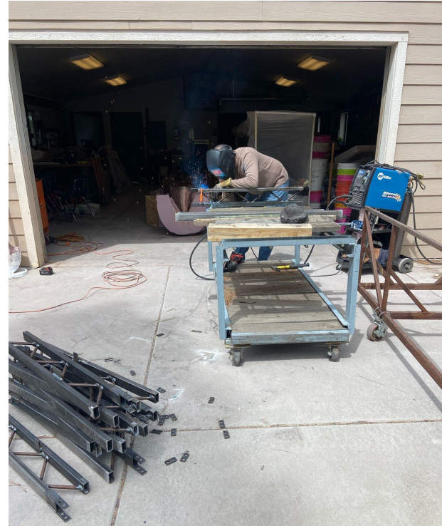
Figure 21, Re-welding Connections
