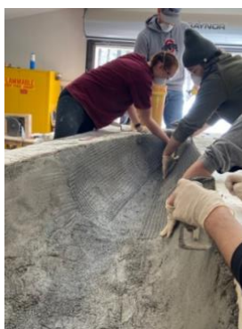
Figure 3-7: Concrete and Reinforcement Placement
