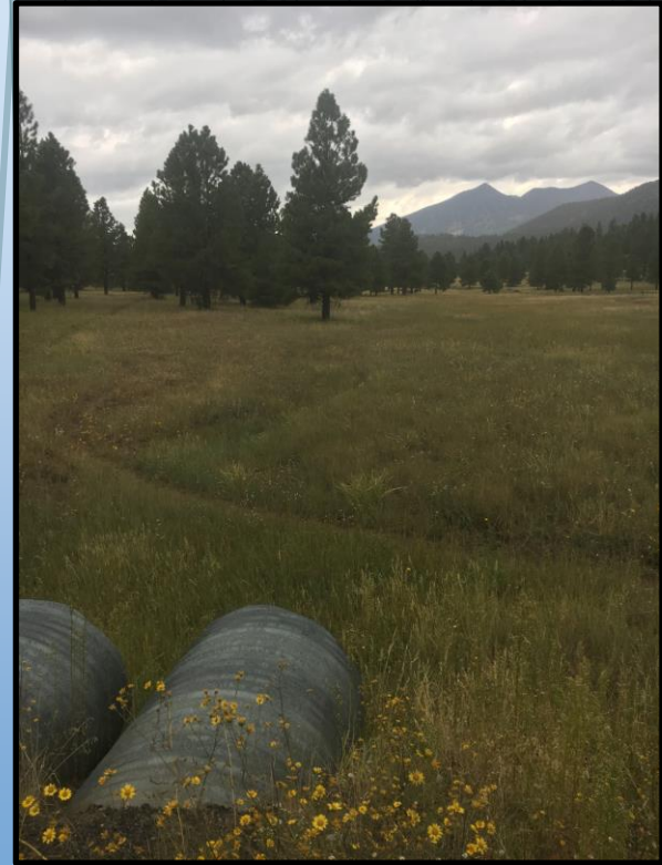
Figure 1: Switzer Canyon Wash Site Visit Photo Credit: Kara Coffel
