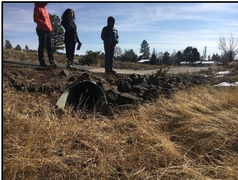
Figure 2.3.6 Inlet of the Culvert Under North San Francisco Street
